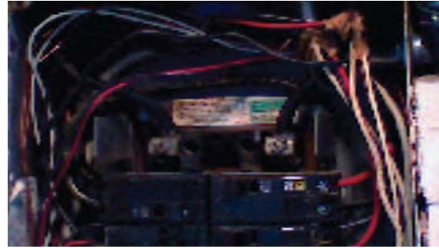
Figure 1 A high-resistance connection or component malfunction within a residential circuit breaker is easily seen in the thermal image, but not in the visible light image.
